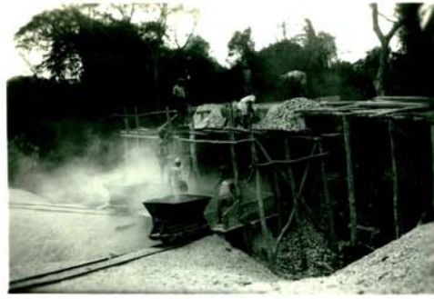
Mowlem Quarry at Bugiri, Uganda, for supply of stone aggregate (chip) for the Tororo to Jinja road, 1954-1955. From top left:- 1. Quarry face with rail bogeys. 2. Stone crusher, with precarious scaffolding. 3. Aggregate (road chip) stacks. 4. Loading out hopper.
