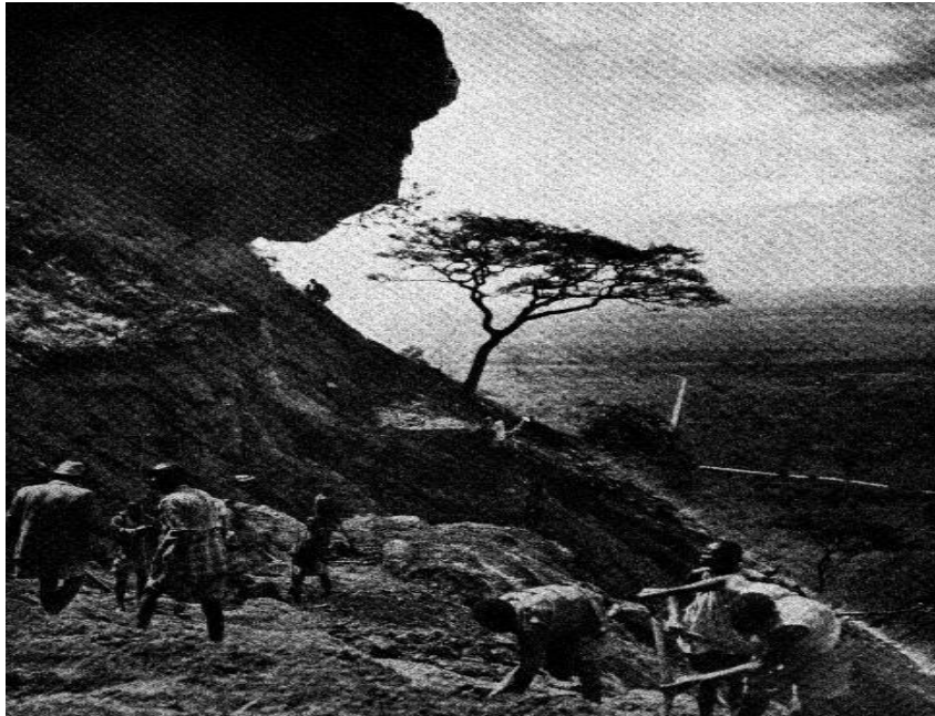
Precipitous Mowlem road building around Mt. Elgon, Kenya/Uganda border, 1956.
