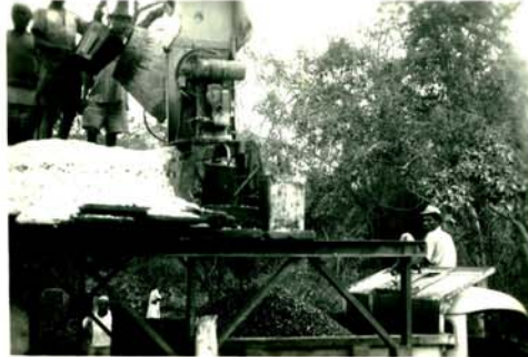
Mowlem Quarry at Bugiri, Uganda, for supply of stone aggregate (chip) for the Tororo to Jinja road, 1954-1955. From top left:- 1. Quarry face with rail bogeys. 2. Stone crusher, with precarious scaffolding. 3. Aggregate (road chip) stacks. 4. Loading out hopper.
