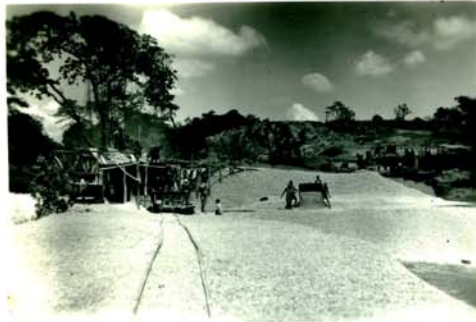
Mowlem Quarry at Bugiri, Uganda, for supply of stone aggregate (chip) for the Tororo to Jinja road, 1954-1955. From top left:- 1. Quarry face with rail bogeys. 2. Stone crusher, with precarious scaffolding. 3. Aggregate (road chip) stacks. 4. Loading out hopper.
