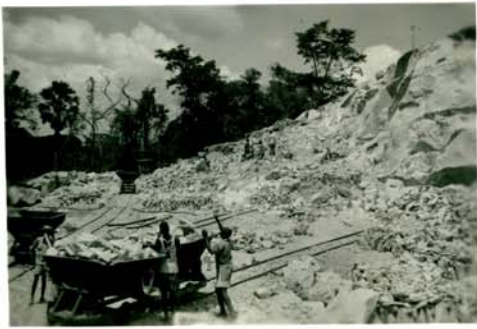
Mowlem Quarry at Bugiri, Uganda, for supply of stone aggregate (chip) for the Tororo to Jinja road, 1954-1955. From top left:- 1. Quarry face with rail bogeys. 2. Stone crusher, with precarious scaffolding. 3. Aggregate (road chip) stacks. 4. Loading out hopper.
